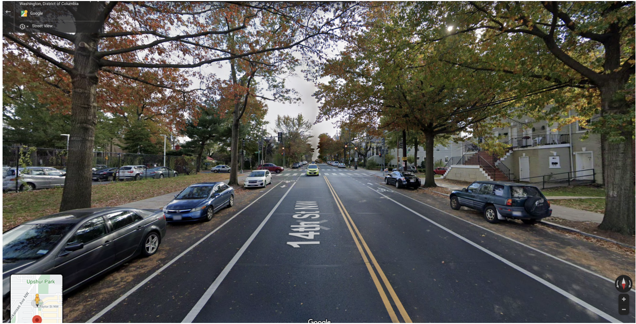
Image 2 Example of 10' wide travel lanes, with bike lanes on 14th St. NW near Taylor Ave, Washington D.C. (12,800 ADT, 2018) 5
